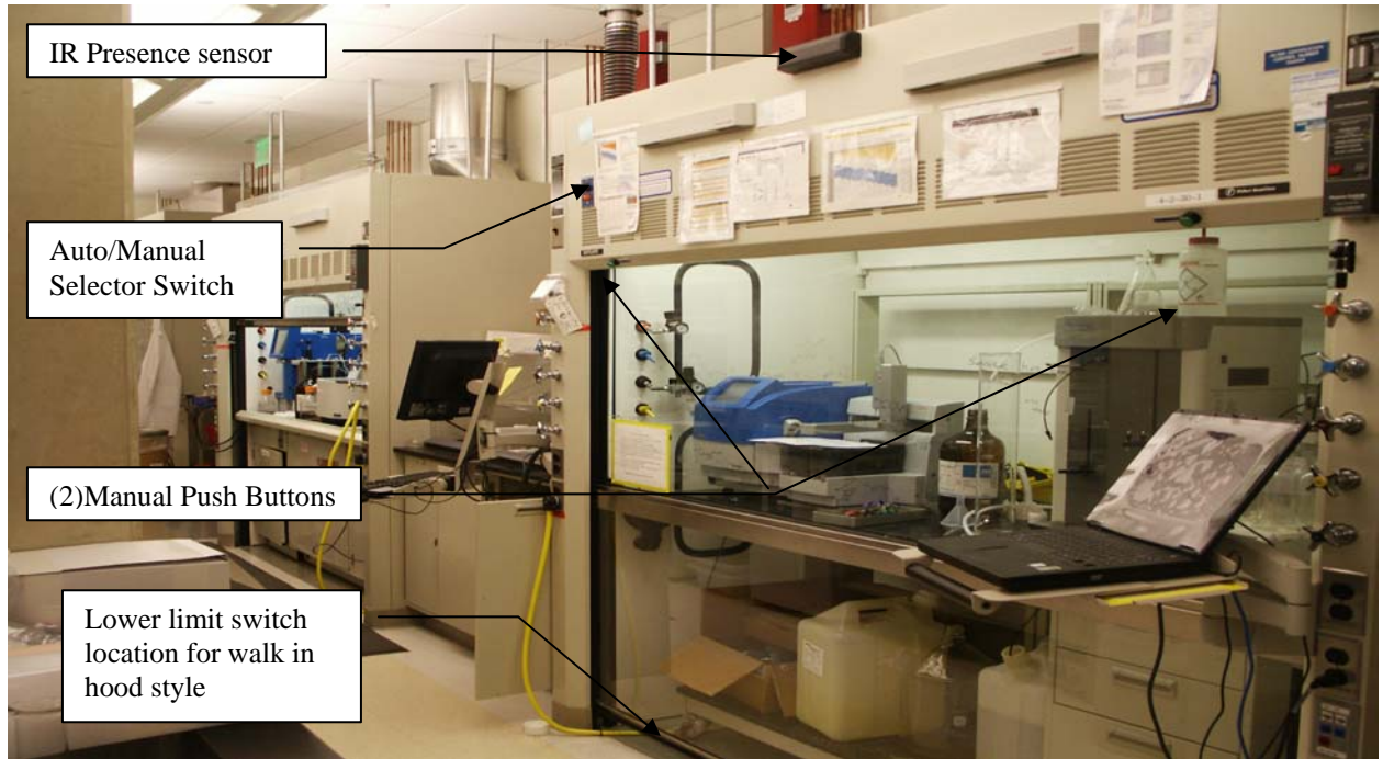
FIGURE 1. FUME HOOD WITH AUTOMATED SASH POSITIONING CONTROL SYSTEM.
