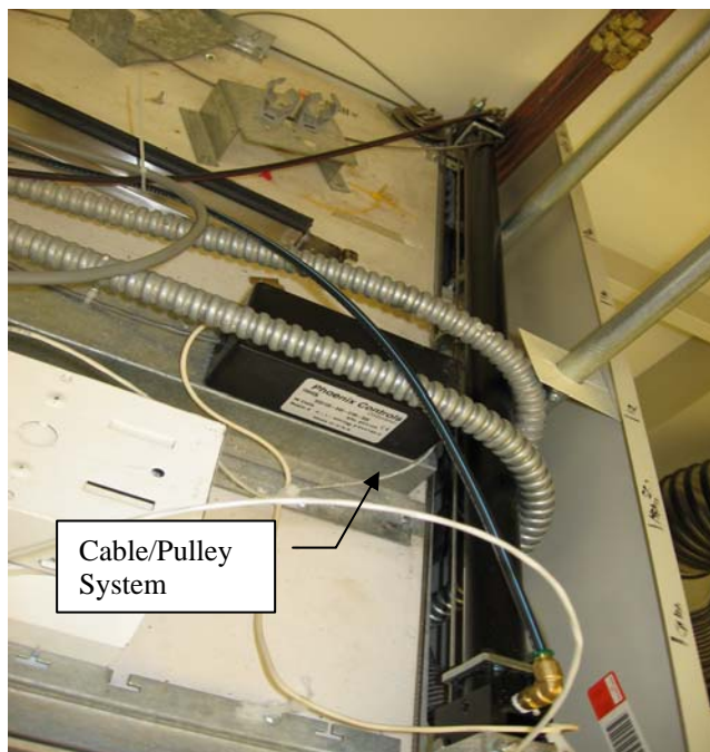
FIGURE 3. THE CABLE/PULLEY SYSTEM ON TOP OF EACH FUME HOOD IS USED TO OPEN AND CLOSE THE SASH TO THE CORRECT, PREDETERMINED HEIGHT.
